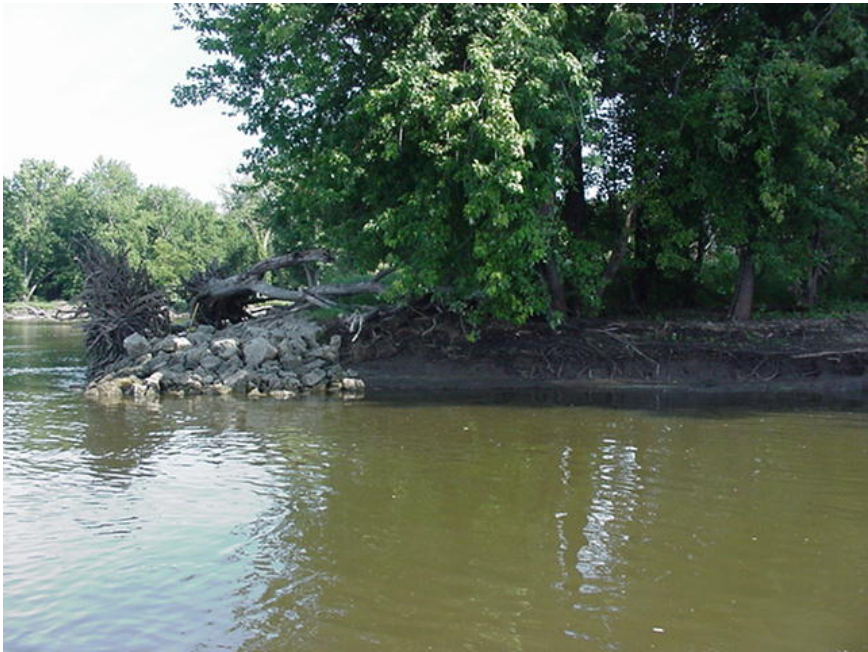
Figure 5 - 10. Bank scour behind downstream riprap protection wing of partial rock closure structure, dated 14 August 2001.
