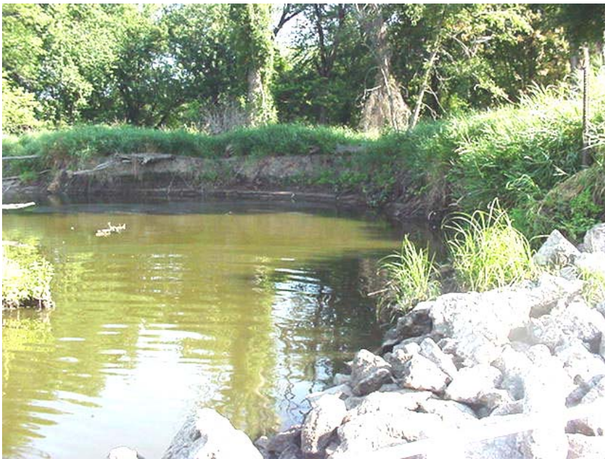
Figure 5 - 8. Bank scour behind left bank of riprap of rock habitat channel, dated 14 August 2001.
