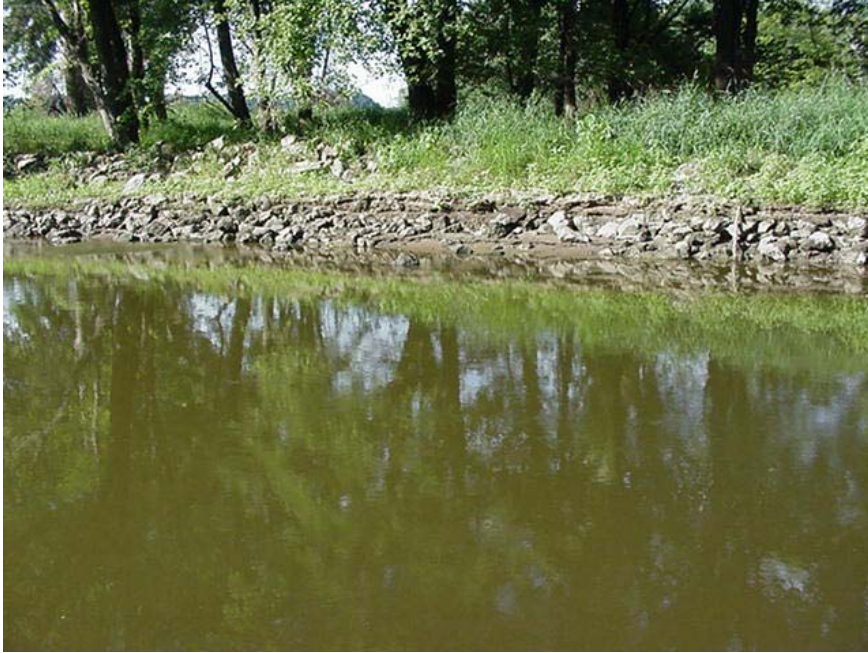
Figure 5 - 9. Sedimentation and scour of rock lined channel, dated 14 August 2001.
