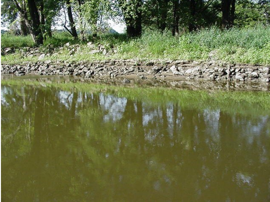
Figure 5 - 12. Sedimentation and loss of riprap to rock habitat embankment, dated 14 August 2001.
