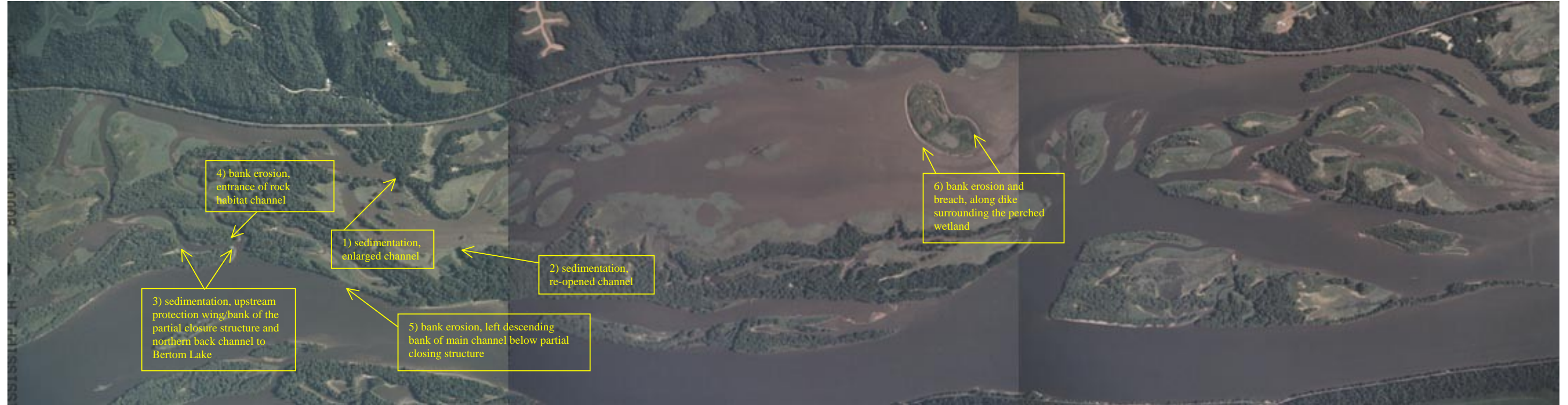
Figure 5 - 15. 2001 Flood Inspection, Areas of Noted Damage noted on 14 August 2001.
