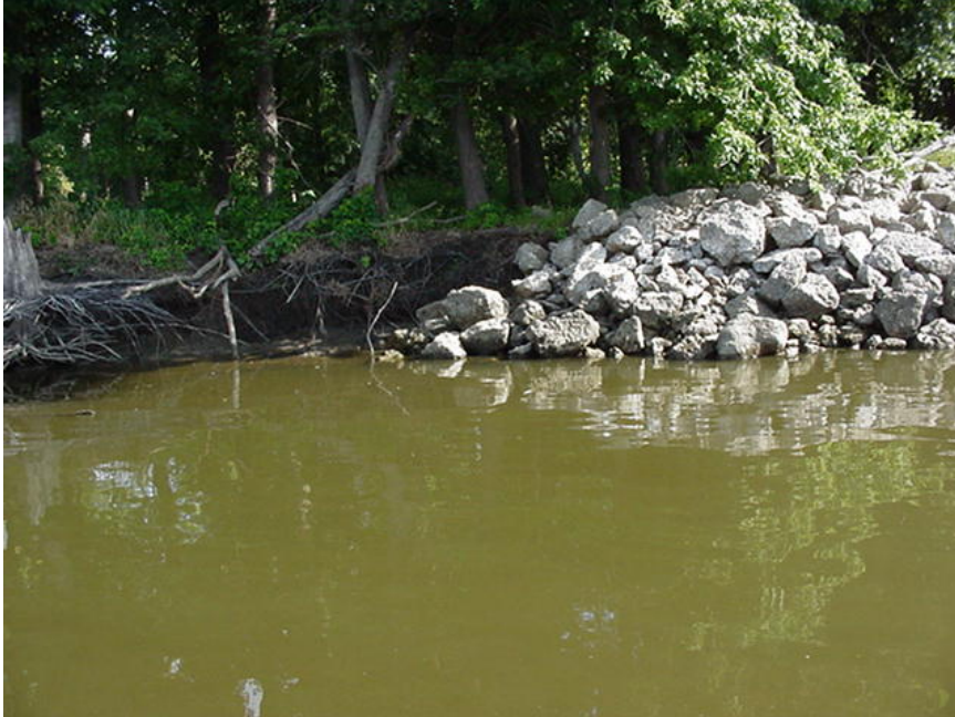
Figure 5 - 11. Bank scour behind upstream riprap protection wing of partial rock closure structure, dated 14 August 2001.
